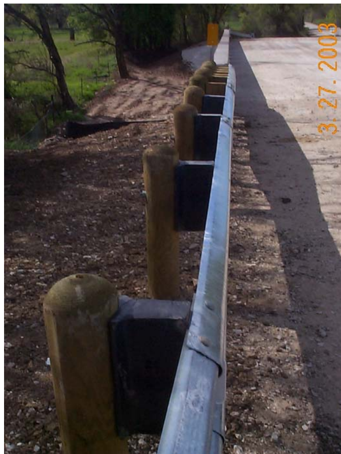
Tire-Rubber Guard Rail Spacer Blocks – TxDOT Brownwood District
