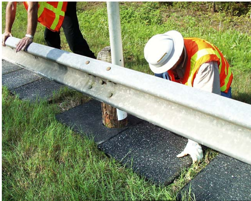
Tire-Rubber Anti-vegetation Mats – TxDOT Lufkin District
