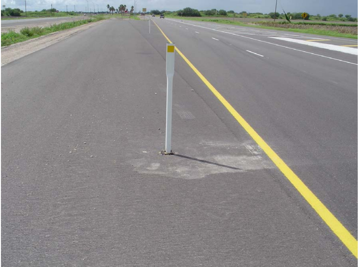
Tire-Rubber Delineator Posts – TxDOT Pharr District
